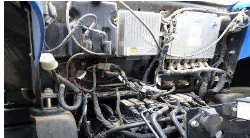
Nav controller mounted outside cab
